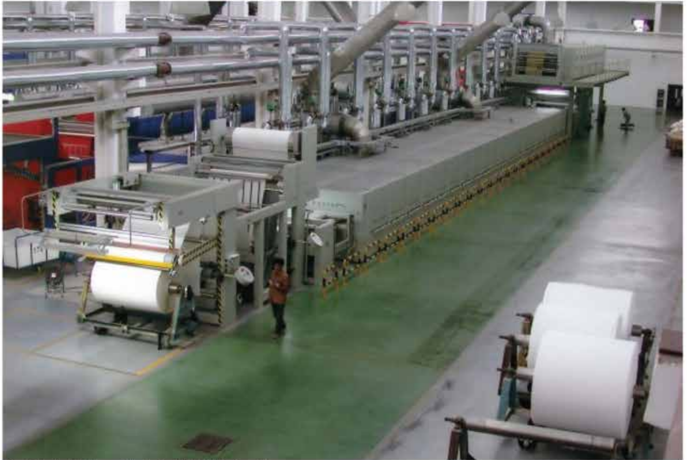
Monforts installation at Lucky Textile Mills in Karachi.
